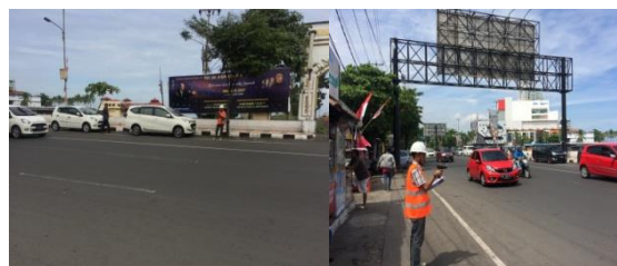
Figure 7. Documentation of Pierre Tendean Street in Manado City (Sta 0+000 - 0+200 Segment).
