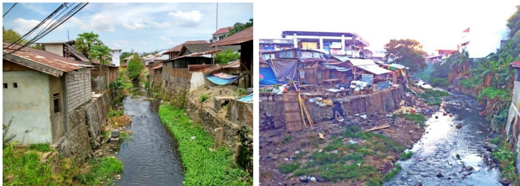
Figure 6. The condition of embankment and river border area in Pinasungkulan Market dan Ranotana Weru Sub District (Segment 1 & 2)
